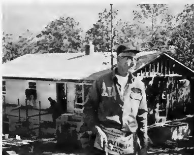
Don Collier, Macon County building site
